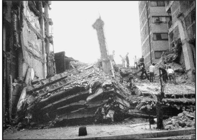
Figure 25 – Only the load-bearing column in the center of the building remained standing after the earthquake.
